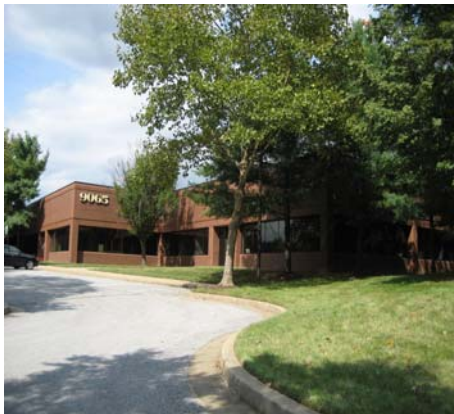
River's Park I & II Columbia, Maryland
