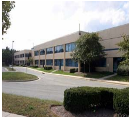
Ammendale Business Park Beltsville, Maryland
